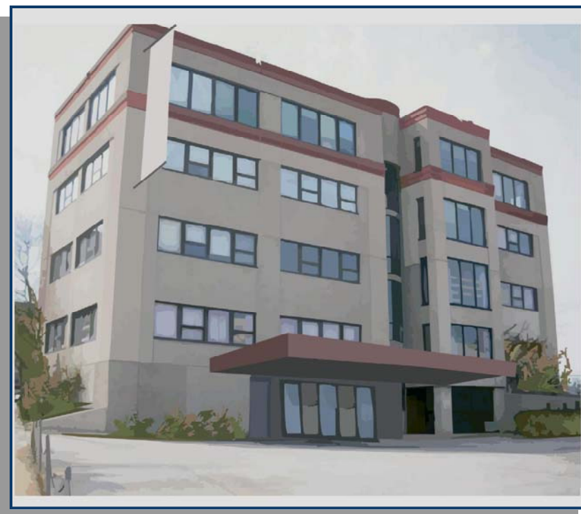
90 Plain Street, 44,000 square foot Class A, Medical Office Building
